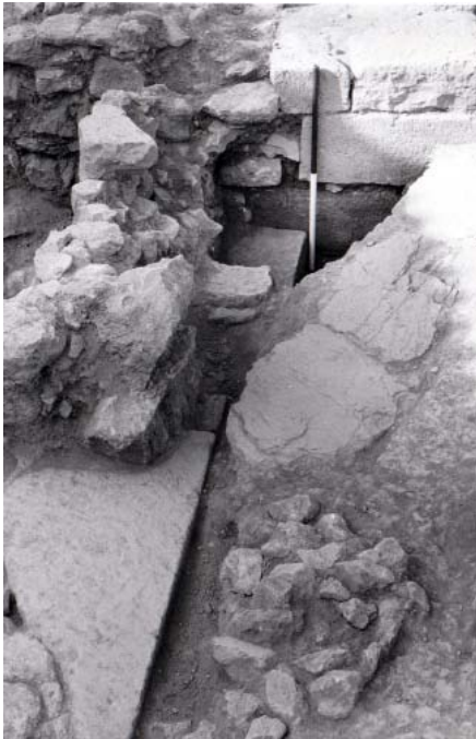
Fig. 12. LM II South House west wall with decayed gypsum top course above LM I A ashlar courses.
