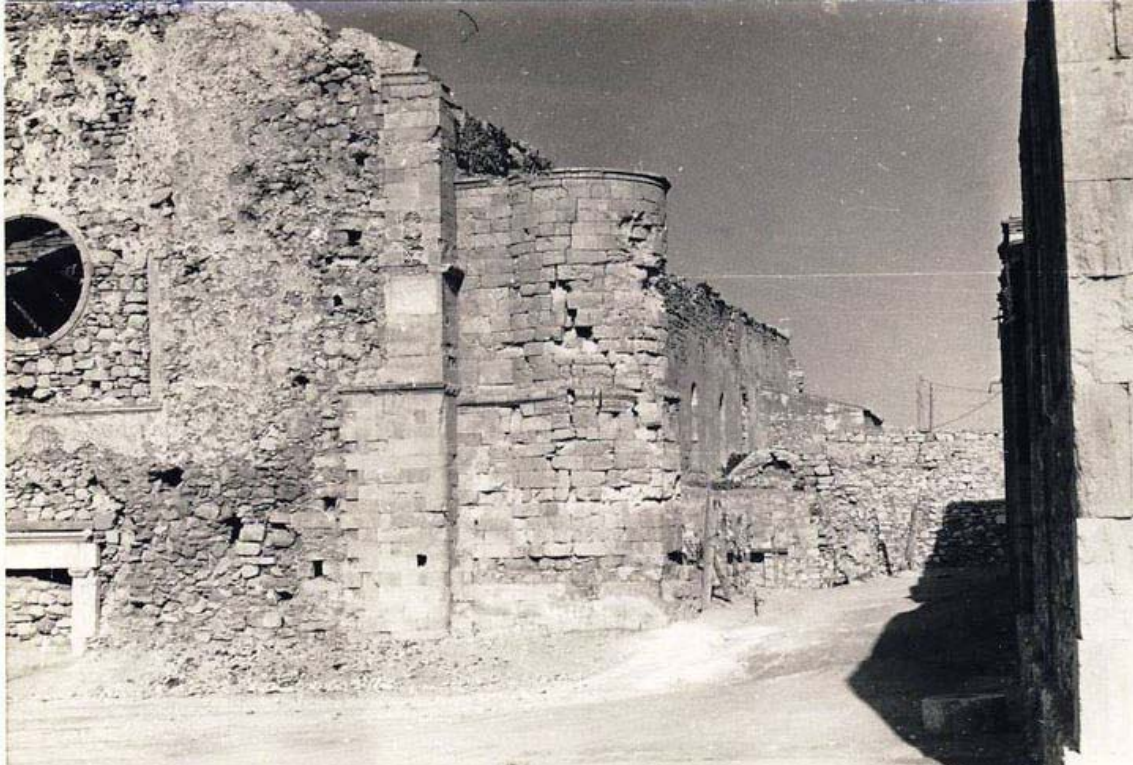
Fig. 3. St Peter of the Dominicans (1970s), before the demolition of the minaret.
