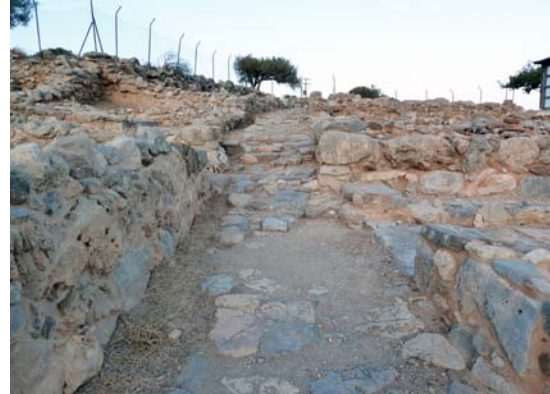
Fig. 5. View of the Harbour Road from the W showing the steps preserved in front of the façades of the buildings and the sidewalk along the north side of the street (Photo by the author).
